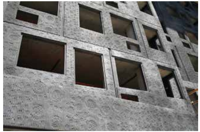
CNC routers are being used to create patterns and grayscale designs by cutting to precise lines and cutting deeper to create a darker tone. Photos: Architectural Polymers.
