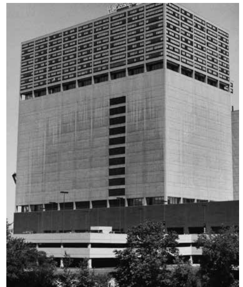
Figure 3 Water washing and dirt deposits.
