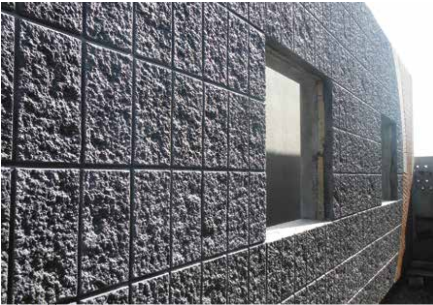
projects, visit www.pci.org/ascent . Textures with significant depth create shadow lines and add aesthetic value to buildings. Photo: Advanced Formliners.
