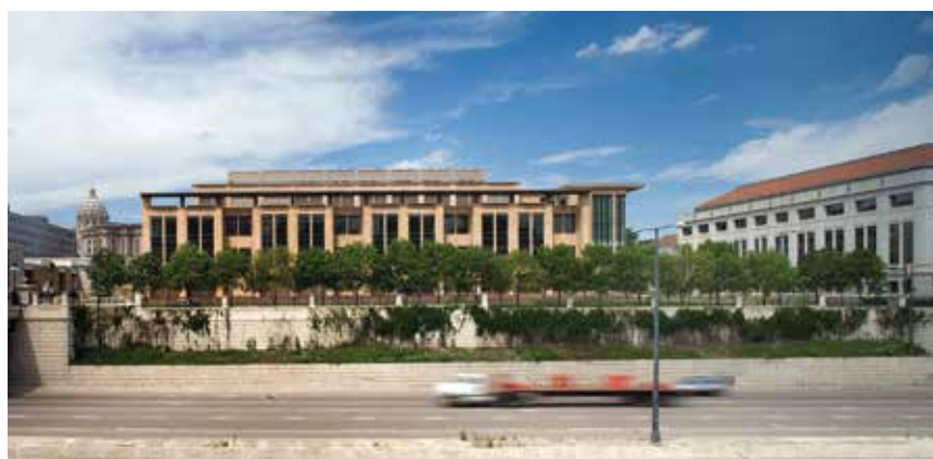
The 176,000-square-foot collocation laboratory for the Minnesota Departments of Agriculture and Health creates collaboration space, as well as clean rooms, laboratories, and office space. The building was clad in architectural precast concrete panels inset with local limestone, which was integrated to conceal panel joints.
