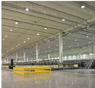
An aggressive schedule and the need to meet strict hygienic standards led designers at this 640,000-square-foot citrus processing and packaging plant in Delano, Calif., to specify a structural precast concrete system including architectural panels.
