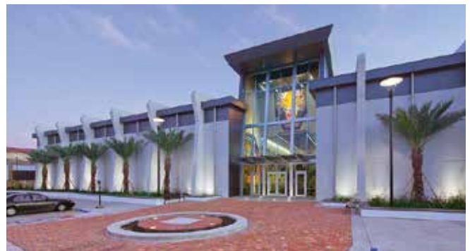
Figure 9 (b) North-facing cladding was a constant mildew-problem—self-cleaning concrete was the solution.
