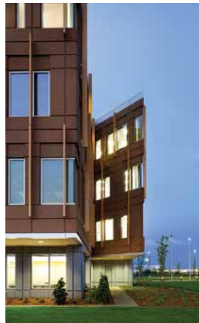
The inspiration for the color palette for this GSA building in Portland, Ore., was the Pacific Northwest and its giant redwoods and sequoias. The precast concrete architectural wall panels feature punched windows in only three sizes to simplify casting. It includes a system of western-cedar patterned, vertical blades applied over the panels to act as sunscreens and reinforce the natural patterns in the landscape. Fine black sand was added to the mix and a light sandblast was applied to achieve the dark
