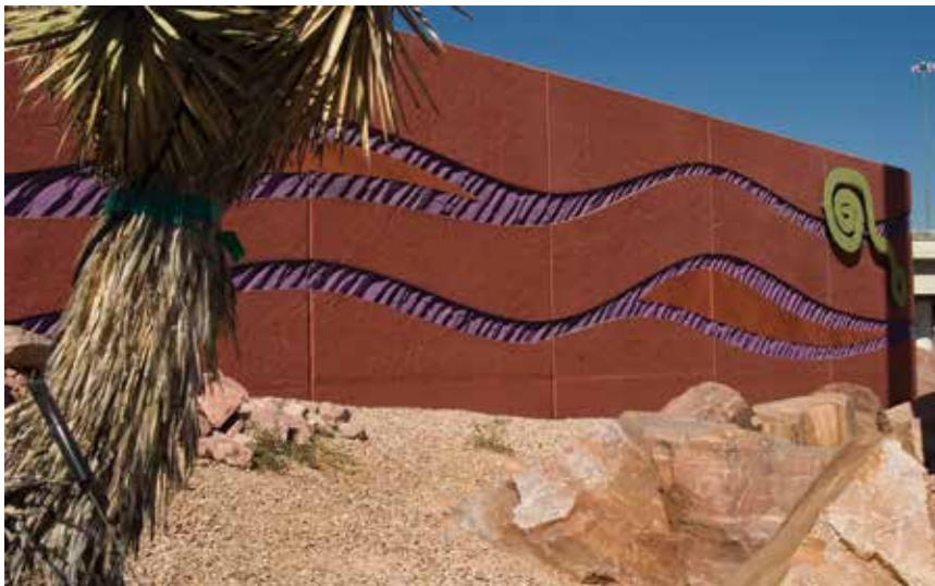
Combining color and forms in a puzzle-piecing type of application can create attractive designs that work well on long surfaces such as soundwalls. This design, which changes every five panels, was created for a Las Vegas soundwall using Rocky Mountain flagstone with bands of purple Oregon Basalt texture, puzzle-piecing the two textures for a continuous pattern along its face. Photo: Scott System.
