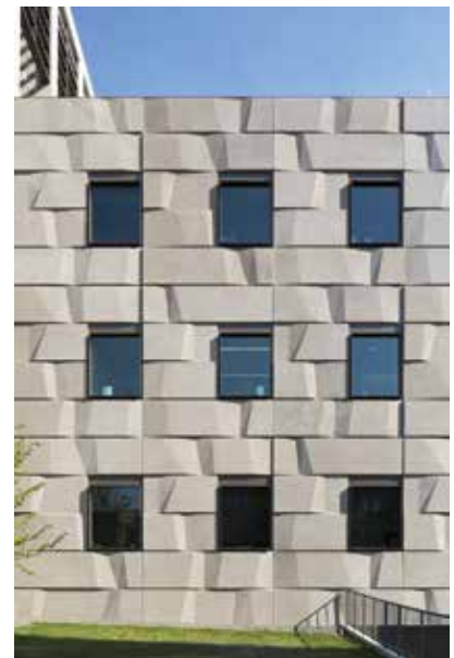
The stone texture on the courthouse's base was created by using 12 formliners combined in different ways, including flipping them 180 degrees, to create larger panels. The panels were erected in a particular sequence to avoid repetition. Each liner had a different skew, creating as much as 4 inches of offset between any two panels.
